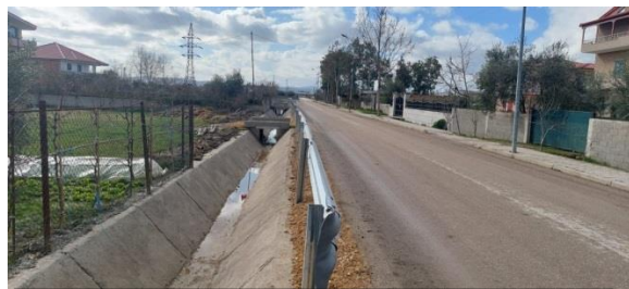
Belina irrigation canal – Jan 2024
