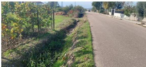
Belina irrigation canal before – Nov 2023
